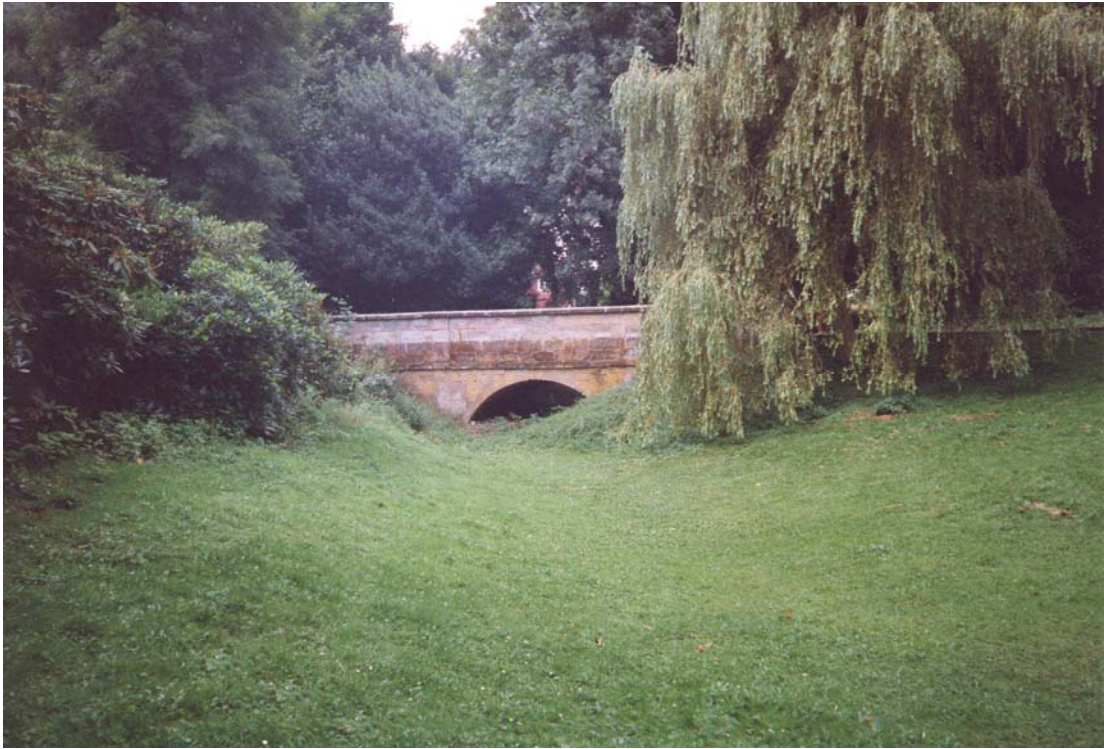
Plate 8 : Angular Bridge over former Church Pool
