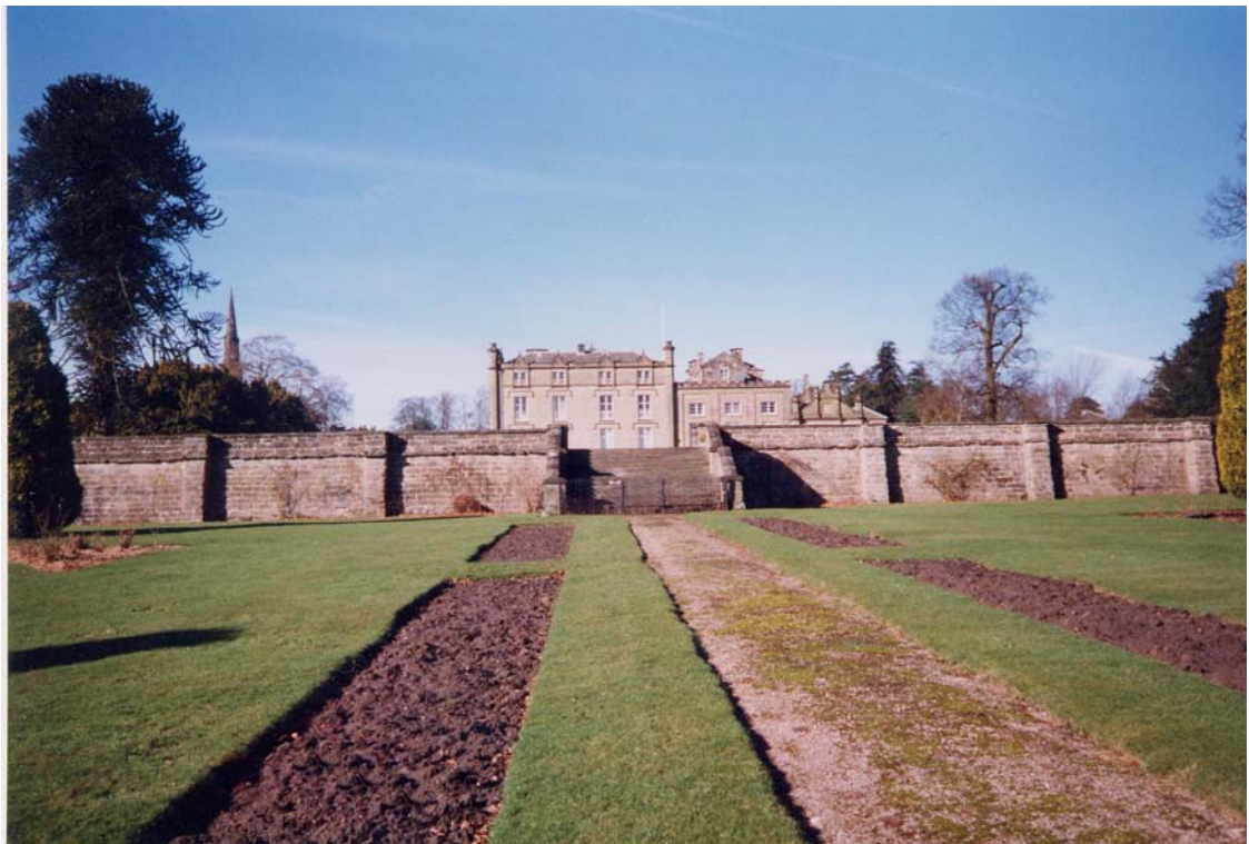
Plate 7 : Terrace Retaining Wall
