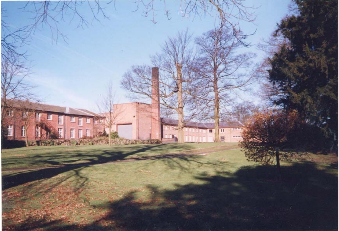
Plate 17 : Post War Office Buildings (Beaumont House) and Boiler House to the North of Coleorton Hall
