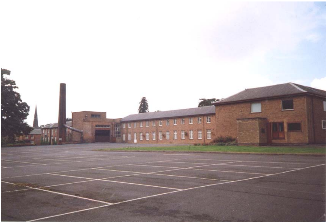
Plate 18 : Post War Office Buildings (Beaumont House) and Car Park to the North of Coleorton Hall
